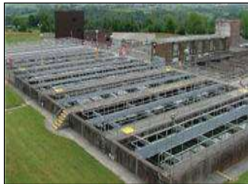
East Waterford Water Supply Scheme
