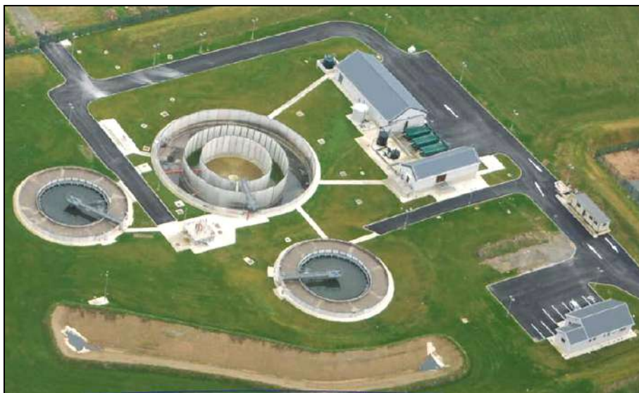
Tramore Wastewater Treatment Plant
